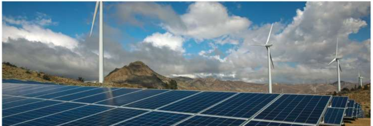
The Pine Tree Wind Farm and Solar Power Plant in the Tehachapi Mountains in Kern County, California is seen in this March 23, 2021 photo. (Photo: Ifan Khan/Los Angeles Times via Getty Images)
