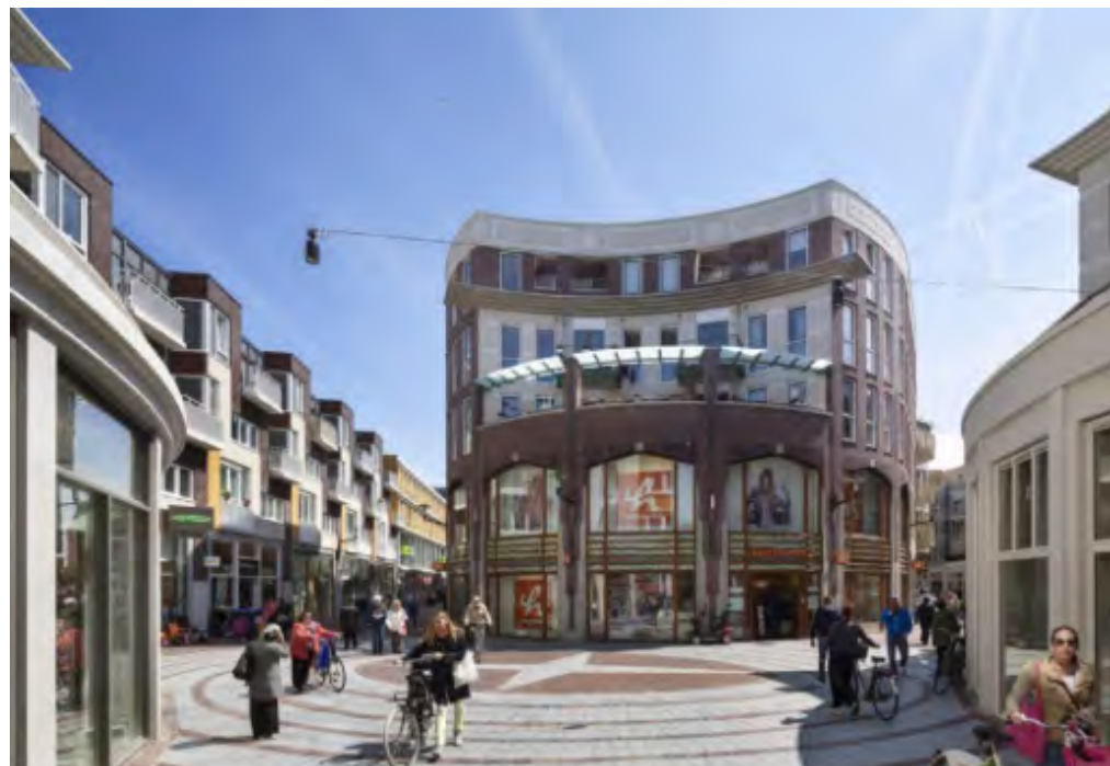
Plein in Oostpoort (Amsterdam) Architect Sjoerd Soeters. Bron: Website van Mollink & Soeters PPHP (Pleasant Places, Happy People).
